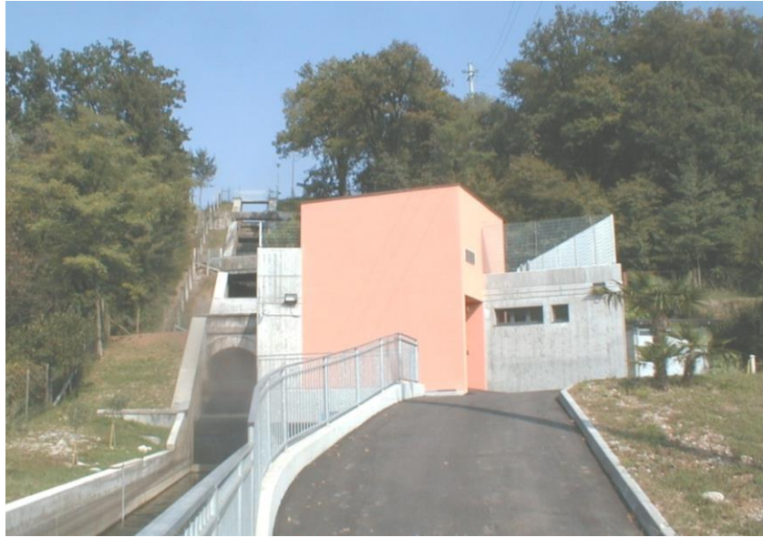
Fig. 4. – Outside of the hydro plant in Esenta seen from the south.
