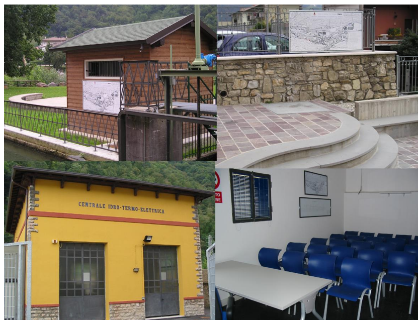
Fig. 3. – Exhibition of explanatory posters in Gardone Val Trompia power plant
