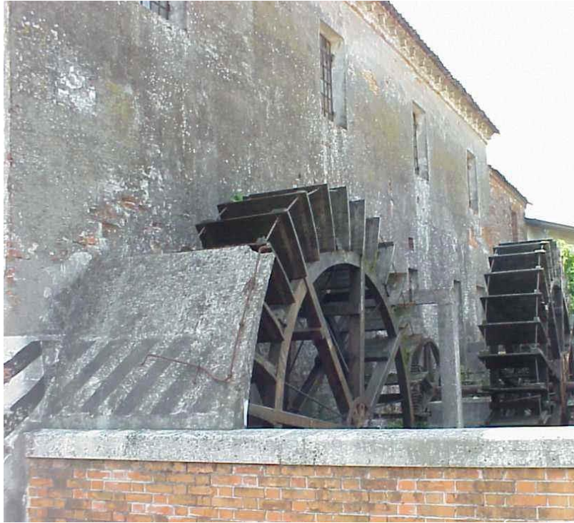
Fig. 1. – Outside of an old mill.
