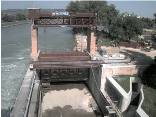
Figure 2 – Module at Chievo Dam housing 5 TG-Units in horizontal configuration. Module shown in lowered position from upstream side, gantry crane to lift Modules, total plant output 1,25 MW
