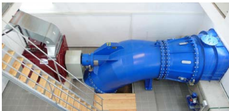
Fig. 3. Example of the horizontal S-Kaplan unit, directly coupled with external generator, like the one in Urago DMV plant.
