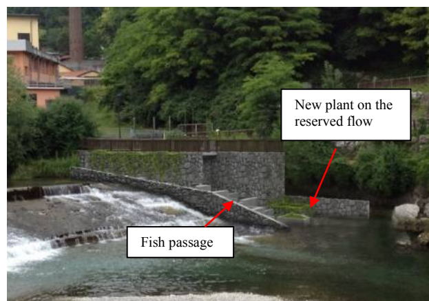
Fig. 1. Casnigo Scarico: the reserved flow plant will be erected at the end of the tailrace channel of the main plant (whose owner is the same of the two reserved flow plants: Casnigo upstream and Casnigo Scarico downstream) adjacent to the fish passage.
