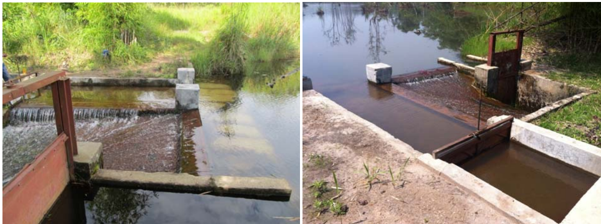
Fig. 5 - Intake structures rehabilitated and upgraded.
