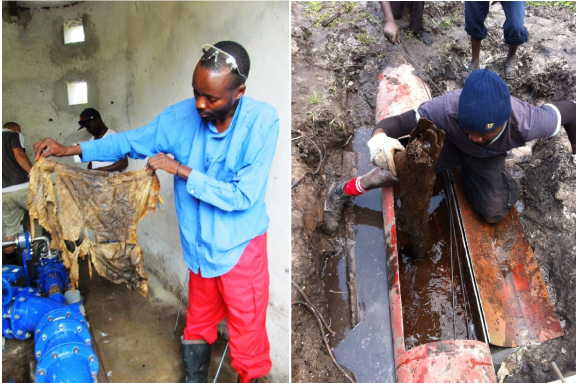
Fig. 13 - Extraneous materials in the penstock ...
