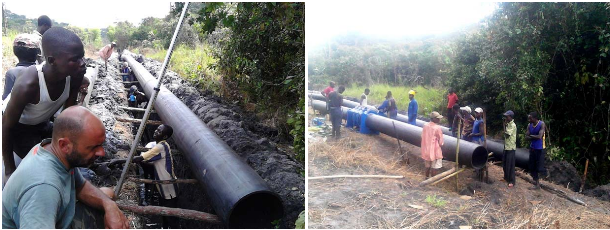
Fig. 10 - Penstock erecting activities.
