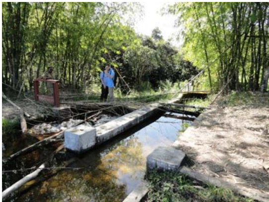
Fig. 3 - Existing intake structure on the Kayoke torrent.
