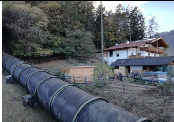
Lana HPP – Private houses close to the penstock
