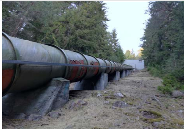
Sarentino HPP – shell conditions
