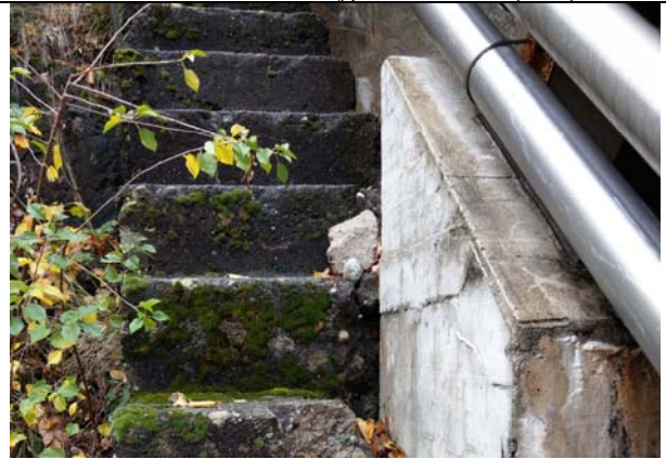
Bolzano EGA HPP – Concrete saddle conditions
