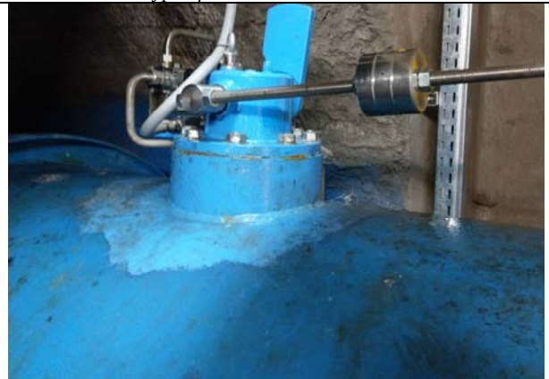
Ponte Gardena HPP – Paddle-Type Flow Switch (D=2)
